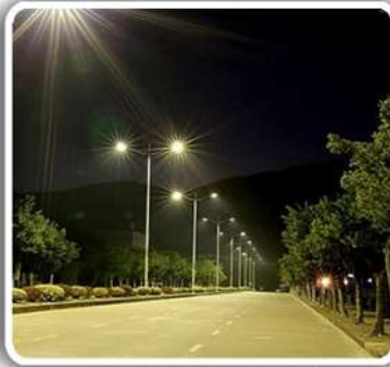
STREET LIGHTS & 24 HOURS ELECTRICITY
